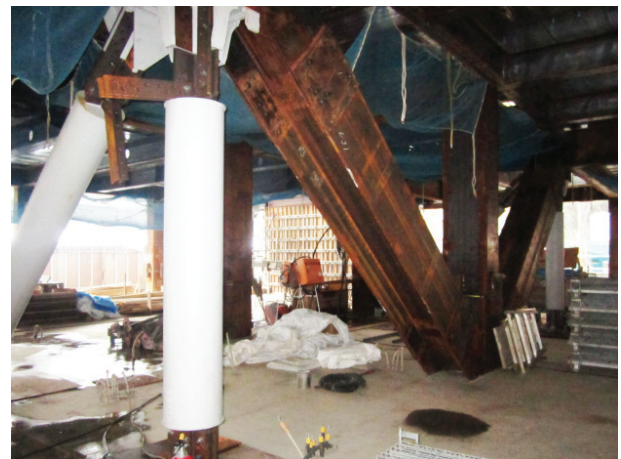
Fig. 18. Construction scene at spine frame.
