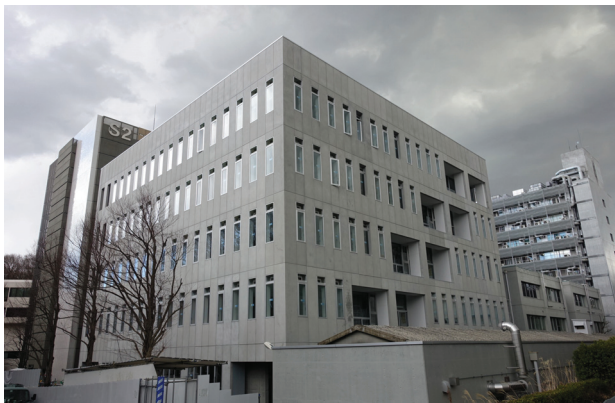
Fig. 14. Tokyo Tech MCES building.
